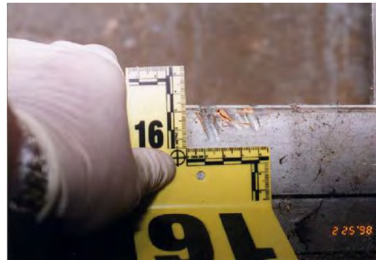
Figure 20 – BCA crime scene photo of south basement window frame
