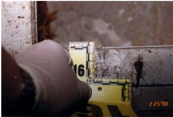
Figure 19 – BCA crime scene photo of south basement window frame
