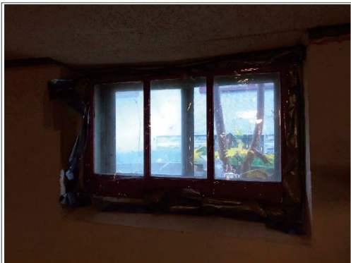
HIS710 – Repair/Rehab Basement Windows
