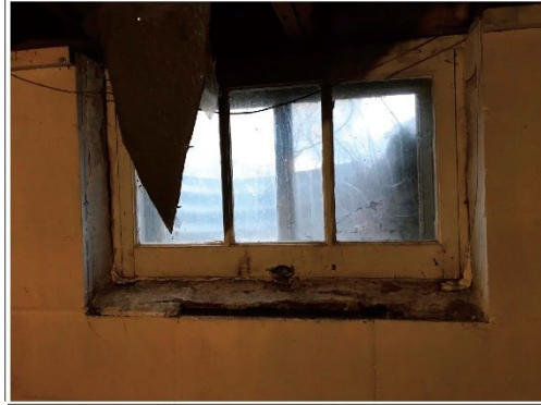
HIS710 – Repair/Rehab Basement Windows
