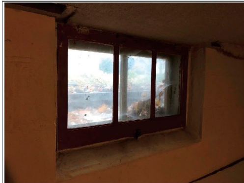
HIS710 – Repair/Rehab Basement Windows
